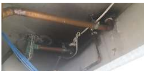
Photo 3 Pipe penetrations through concrete slab.
