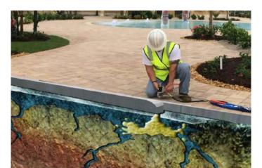
Expanding polyurethane (PU) resin injection technology is primarily used for slab jacking. It raises, corrects and strengthens moving and sunken concrete structures on, or in, the ground.
