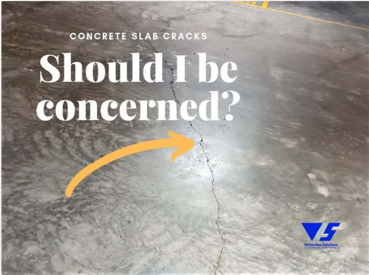
Photo 6 Concrete Slab Cracks - Should I Be Concerned? - Waterstop Solutions
