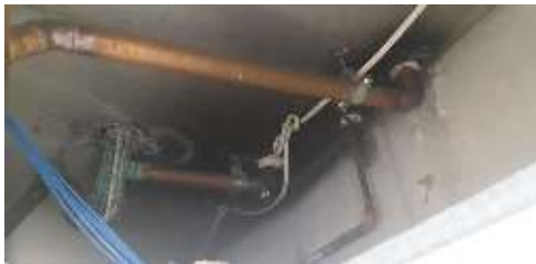
Photo 3 Pipe penetrations through concrete slab.
